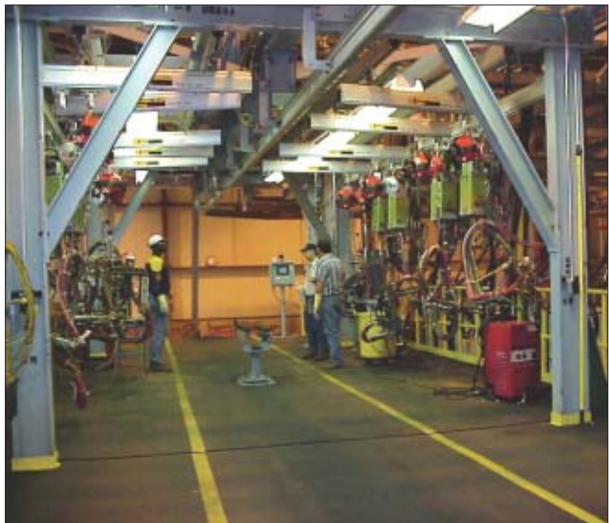
Ingersoll-Rand rail system application shown in a manufacturing facility.
